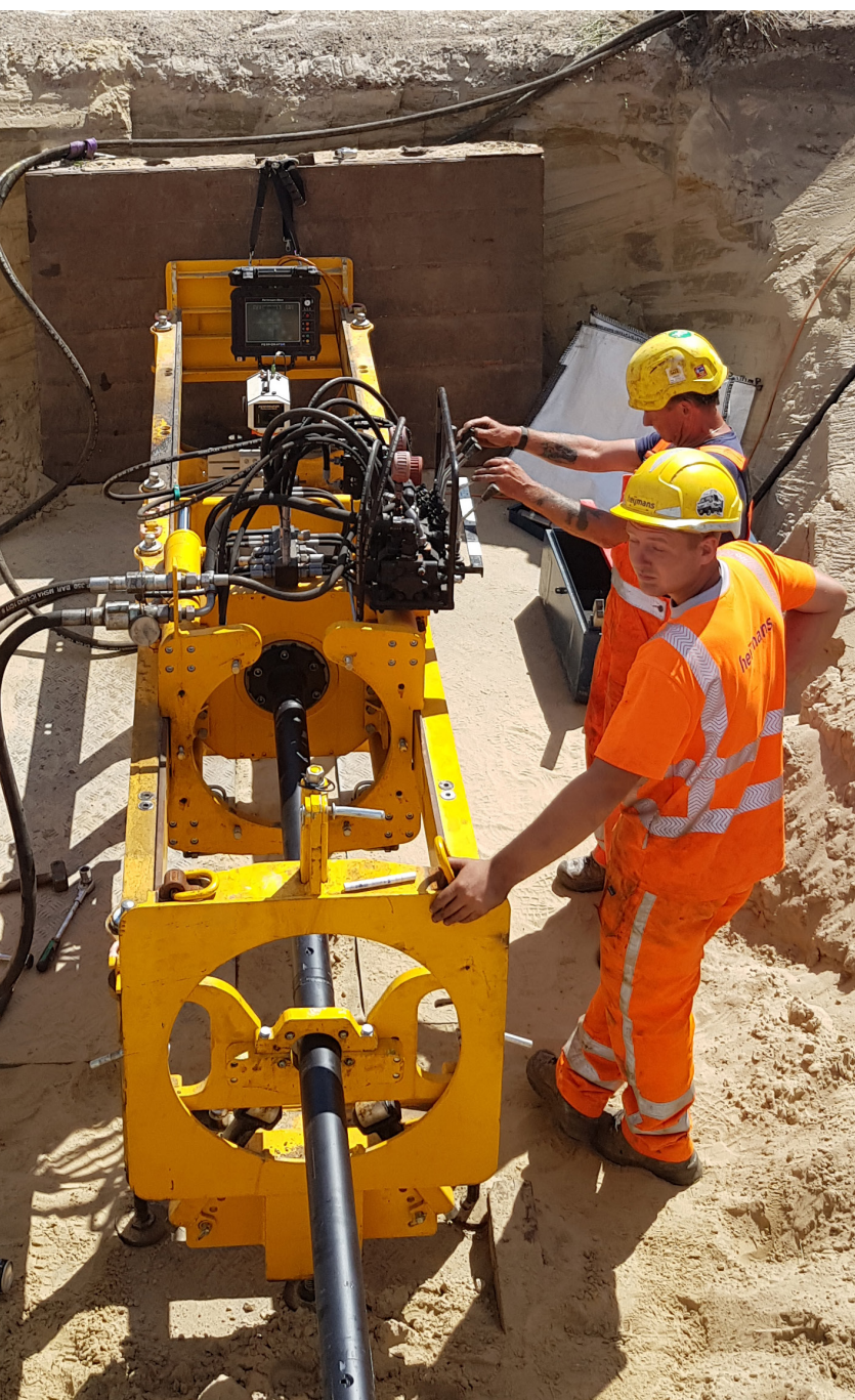
Pressbohranlage / Auger Boring Machine PBA 40N
